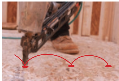
Bump firing or bounce nailing is using a nail gun with a contact trigger held squeezed and bumping or bouncing the tool along the work piece to fire nails. Red dots show path of motion.
